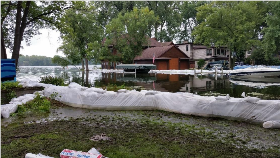
Figure 3 – Sandbags placed to alleviate flooding in Monona, WI
